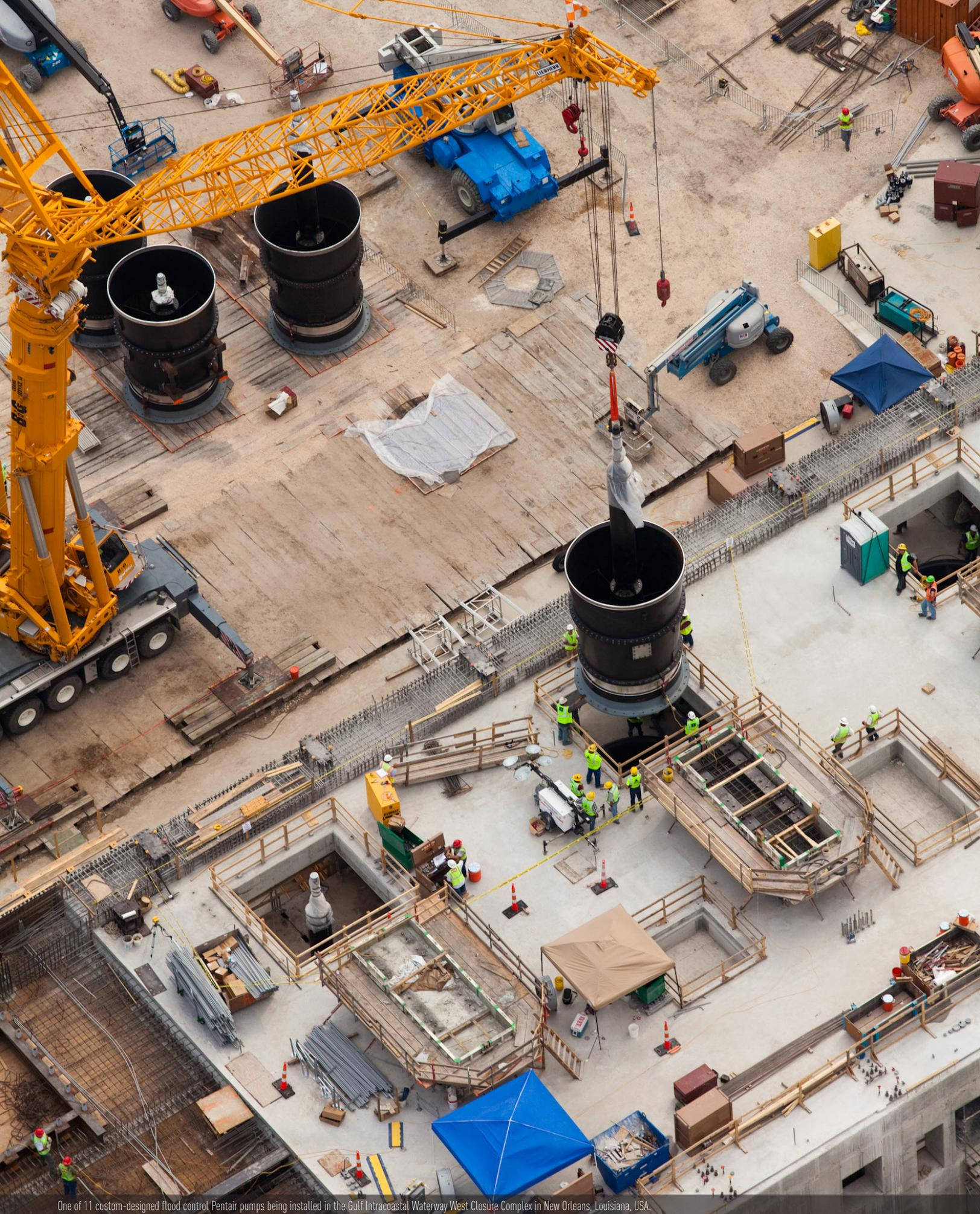
One of 11 custom-designed flood control Pentair pumps being installed in the Gulf Intracoastal Waterway West Closure Complex in New Orleans, Louisiana, USA.
